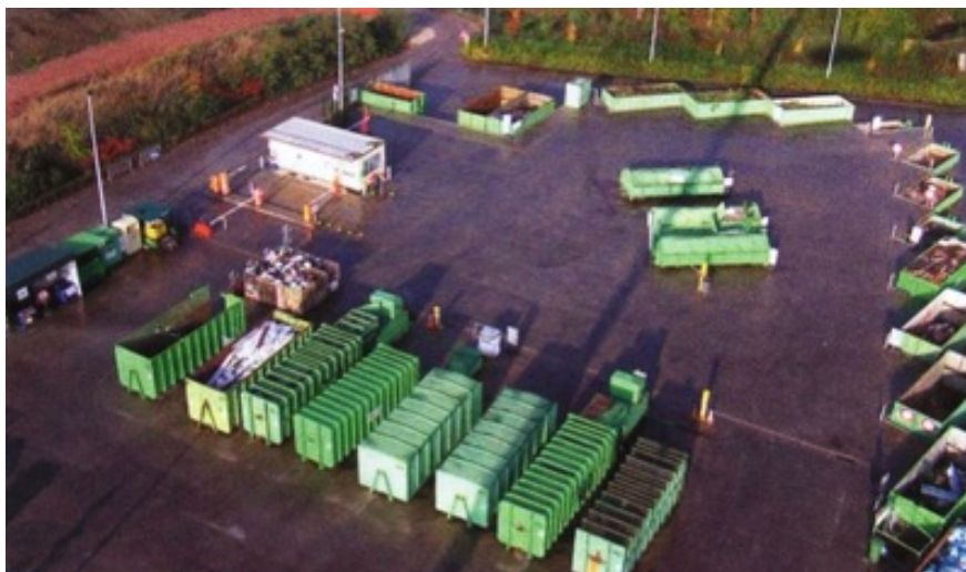
Figure 6: Waste collection yard
